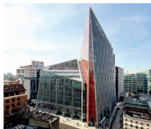
Work and play at Nova, SW1 – completed in April 2017.
