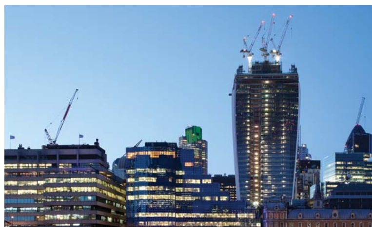
20 Fenchurch Street, EC3, taking shape
